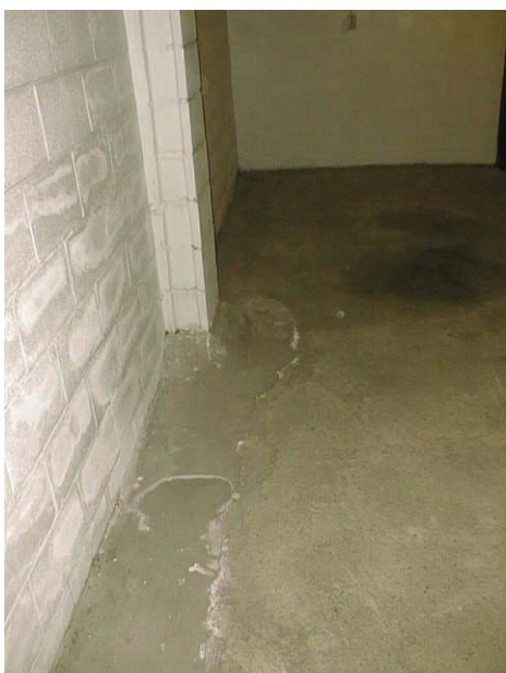
Photo 9 , Example of where concrete was removed and drain was installed.
