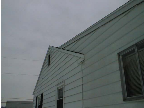
Photo 1 , Roof line where addition adjoins the house.
