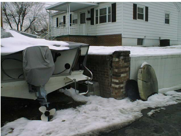
Photo 14 , Neighbors end of retaining wall.
